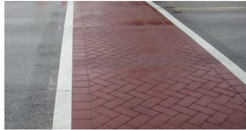
Crosswalks enhanced with color and texture draw drivers' attention and make crossing safer. Source: www.westchicago.org
